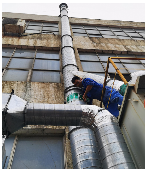
废气排放口标牌
